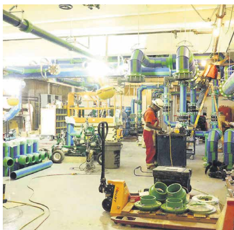
The SFU data storage hub (here under construction) is part of the infrastructure of advanced computing, storage and software solutions that accelerate research and innovation. SUPPLIED
