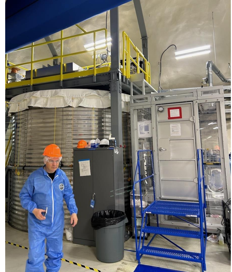
CUTE Test Facility is an example of a facility transferred to SNOLAB ownership.
